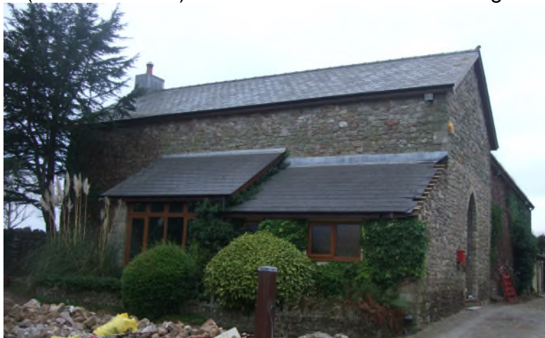
Front (north elevation) and eastern side of the existing building
