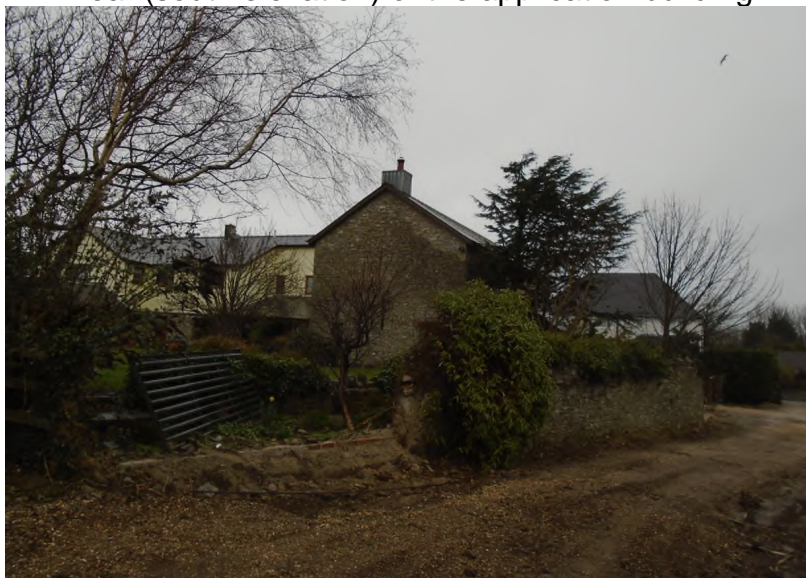
Rear (south elevation) of the application building
